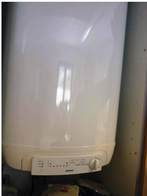
Abb. 22: 80 l-Warmwasserboiler
